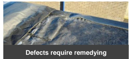
PVC Single-ply roof
