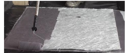
Wetting through the fibreglass CSM
